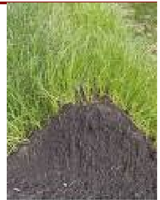
Seeded compost berm
