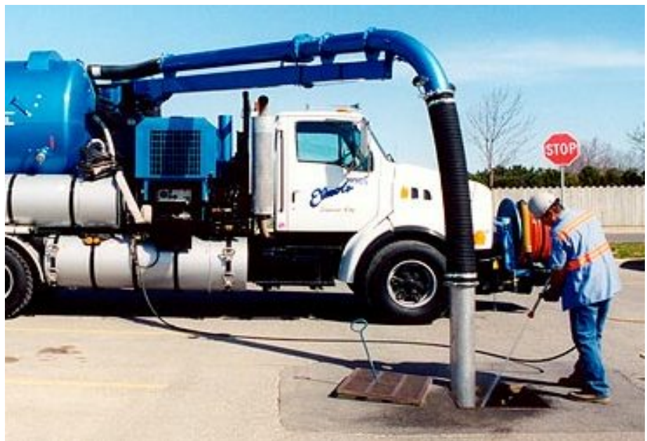
Vac truck cleaning out storm drain
