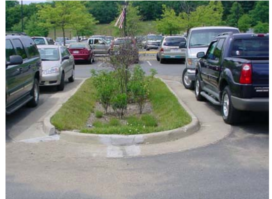
Infiltration islands in parking lot
