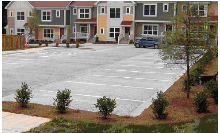
Pervious concrete and infiltration basin captures the 2-year 24-hour storm
